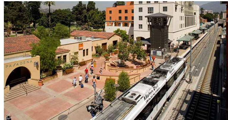
Del Mar Station, Gold Line | Pasadena, CA
