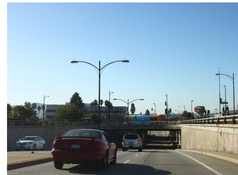
Hollywood Way underpass at Empire Avenue.
