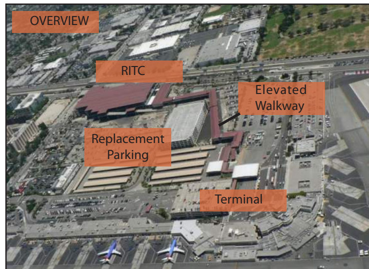
Overview of the recently completed RITC
