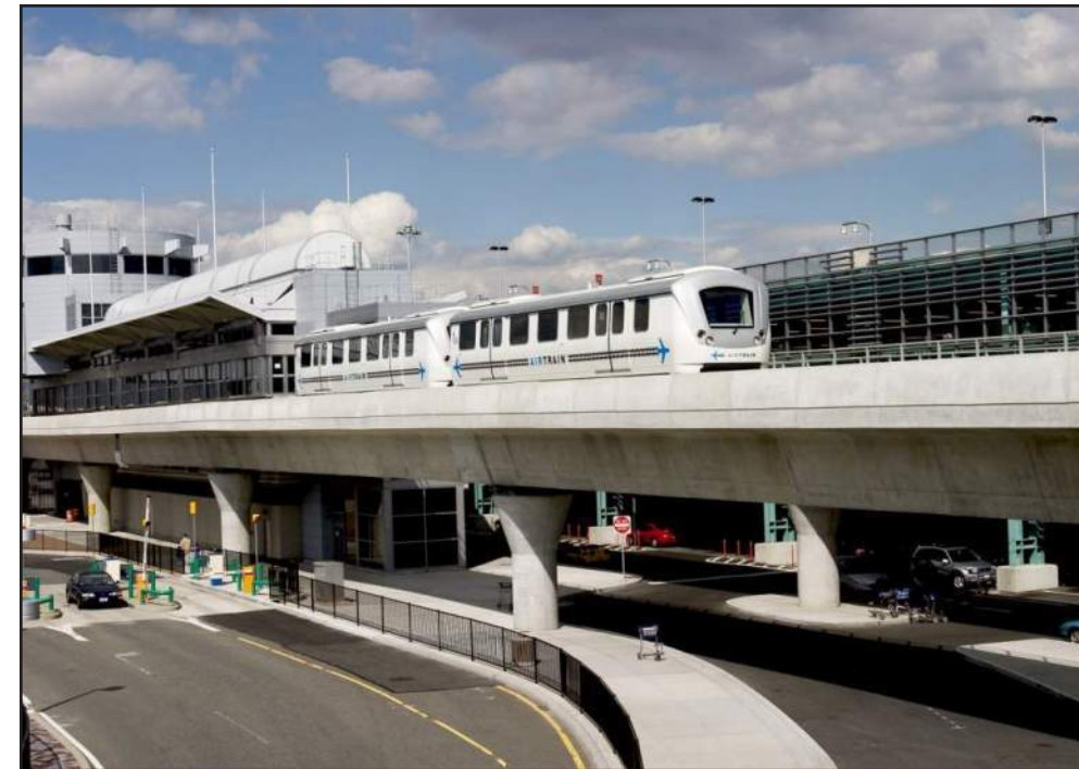
Airport Automated People Mover
