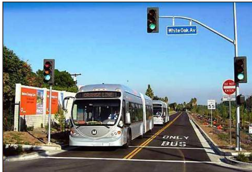
Existing Metro Orange Line bus in dedicated busway
