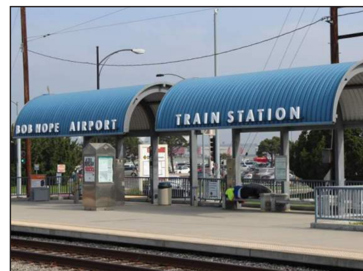
The existing Bob Hope Airport Metrolink Station
