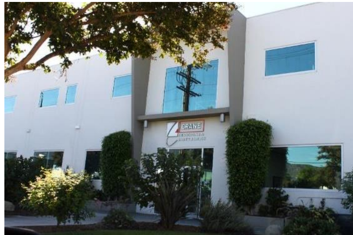
Example of existing industrial and commercial use
