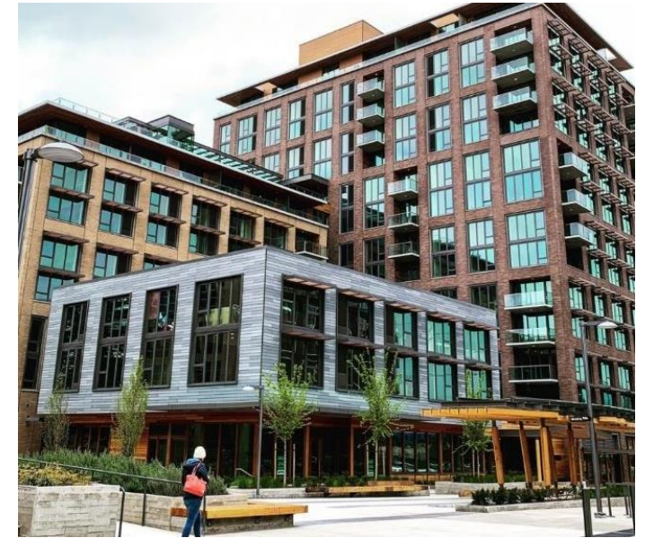
Example of twelve story mixed-use development with gradual transitions to the street
